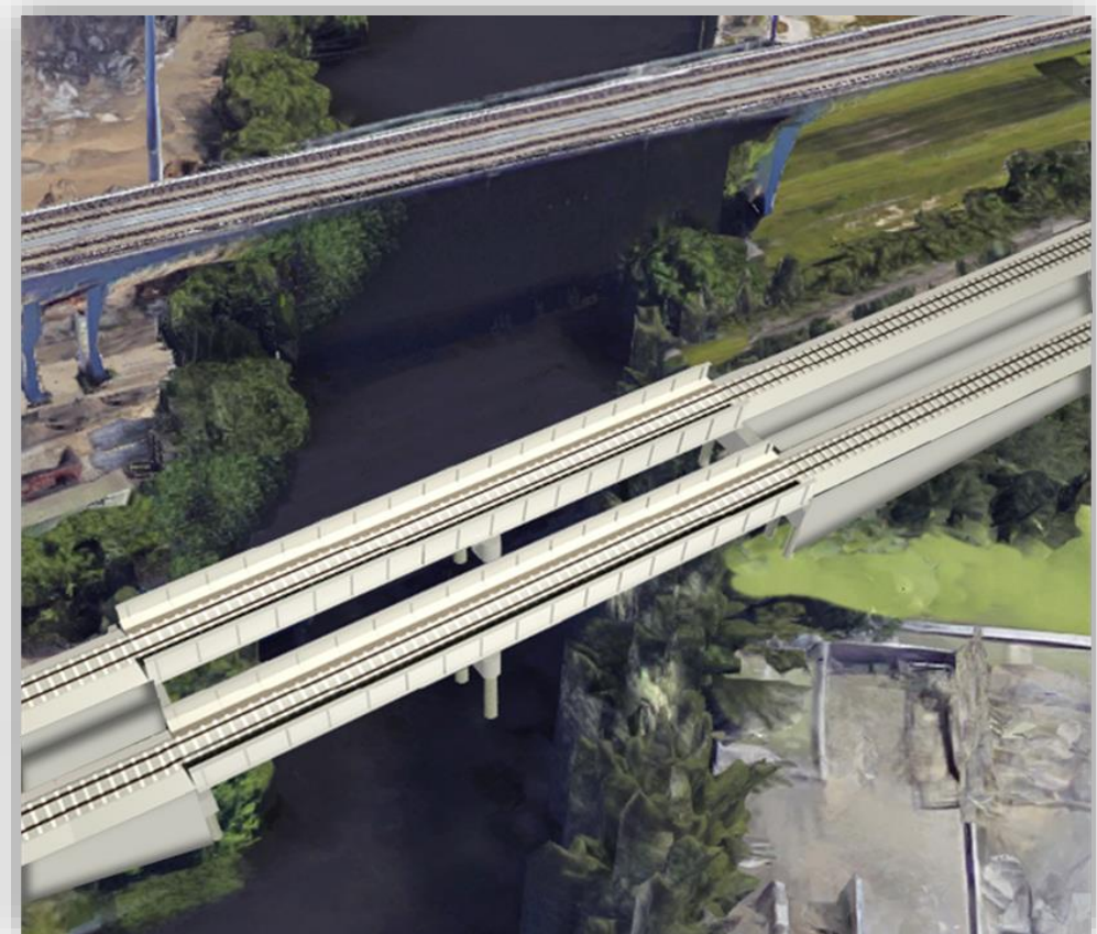
Proposed – Two single track fixed bridges
