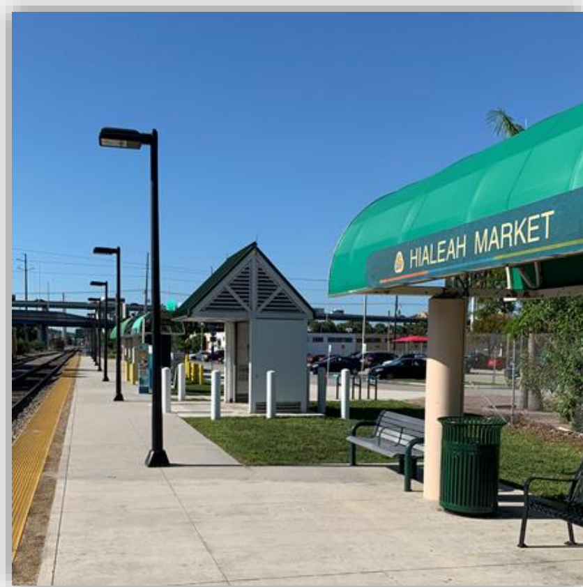
Existing Station – West Side Platform
