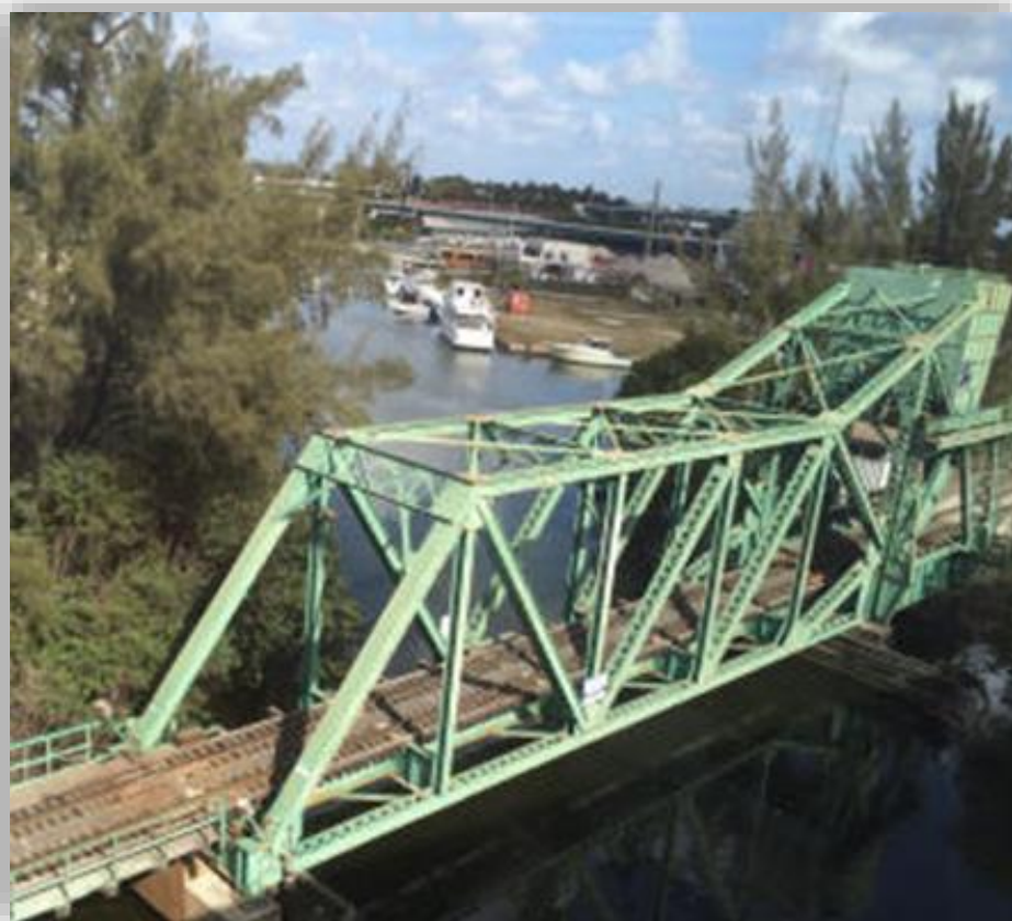
Existing Single Track Bascule Bridge
